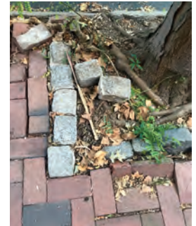
Loose Belgian blocks around a tree pit are a tripping hazard.
